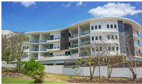
42 Gothenburg Crescent, Stuart Park
